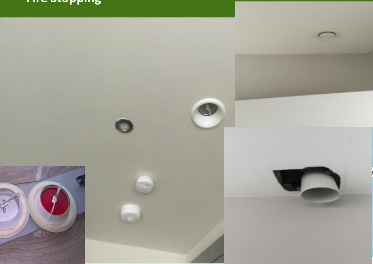
Fire Rated Ceiling Air Valve sealed after a fire
