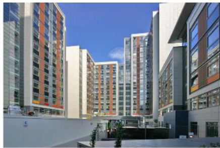
'Paragon' 17 storey volumetric modular building – evacuated
