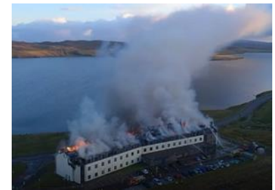
Shetland SIPS modular hotel fire
