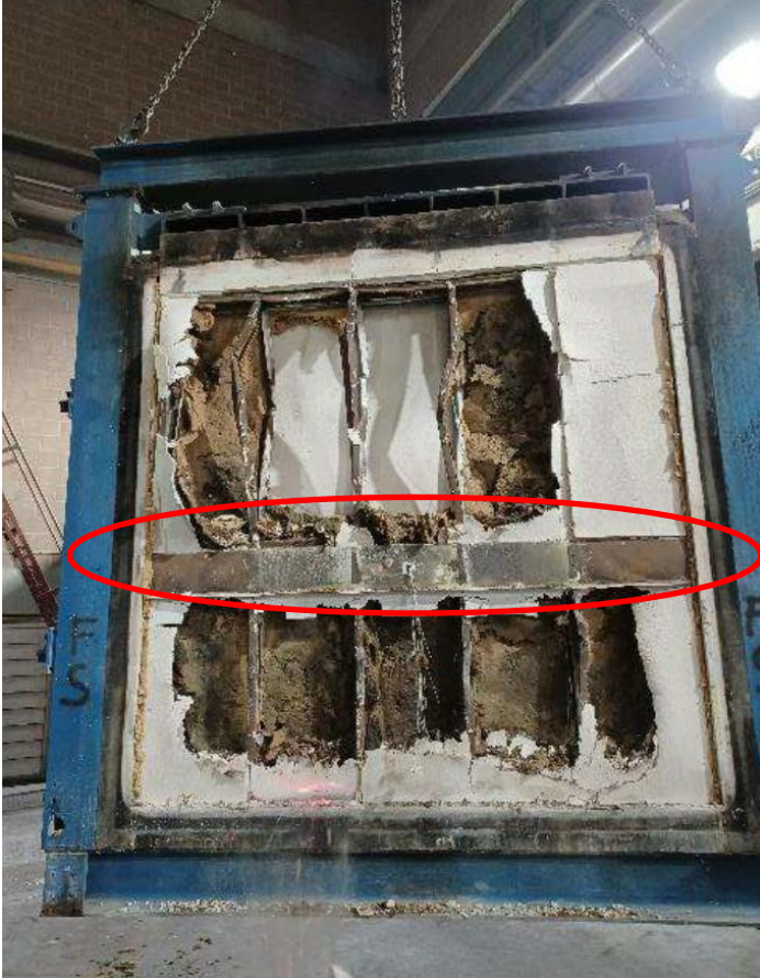
Post test exposed side wall panel (source: Evolusion Innovation)
