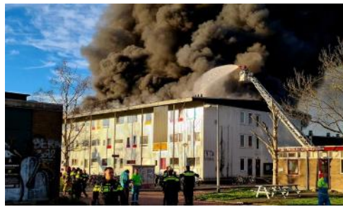
Amsterdam apartment volumetric modular building – demolished post fire
